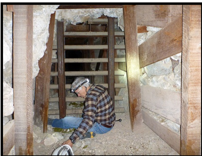
Figure 15. Bat compatible gate at Crackerjack 14 Mine.
