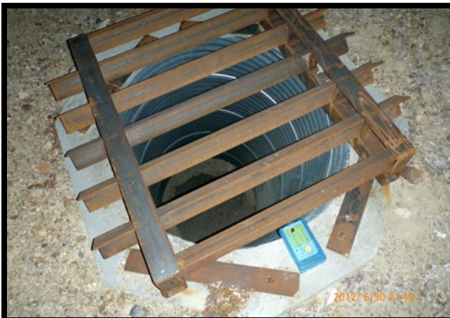
Figure 14a,b &c. Goldstone Mine. A cupola (a) and a dangerous stope (b) at main mine #43, and a vertical metal culvert (c) at Goldstone #42a that is not a bat compatible closure.
