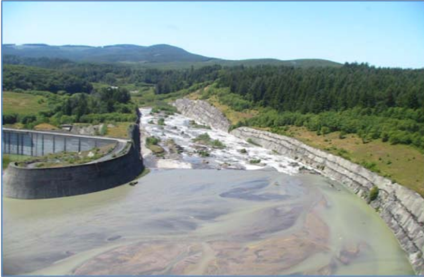
Figure 3.7 SRS Spillway Looking Downstream
