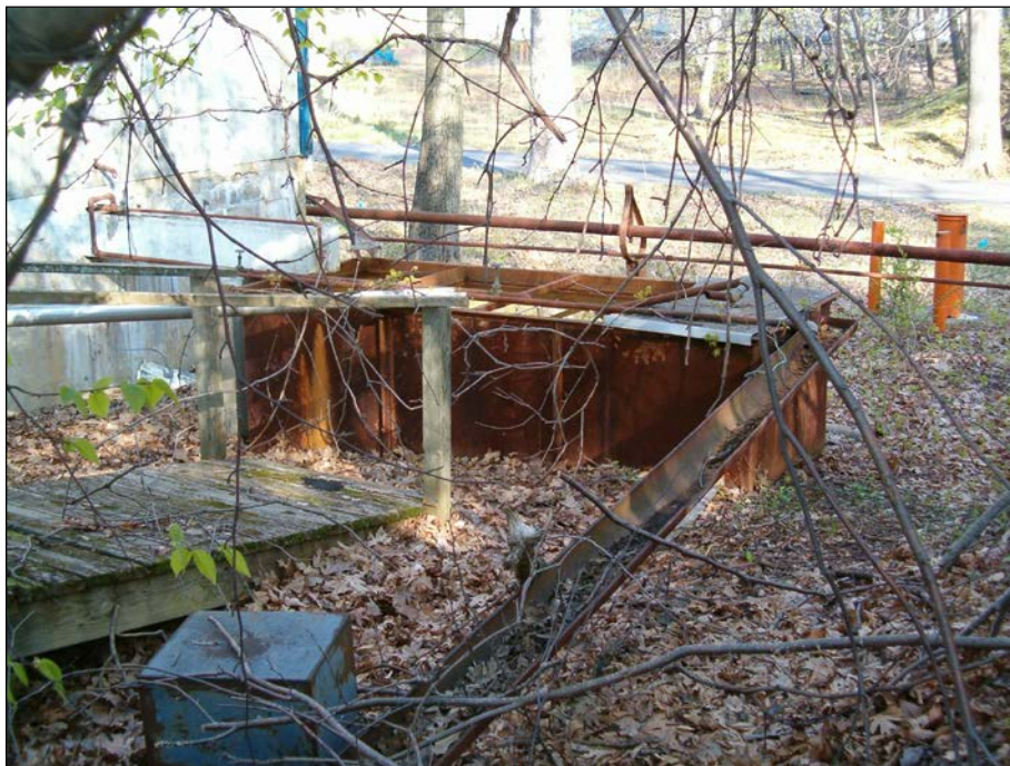
Figure 4.5. Collection boxes for wastewater and washdown water located northeast of Building 823 in Area 157.
