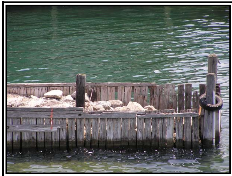
Figure 7 – Condition of the Eastern Breakwater
