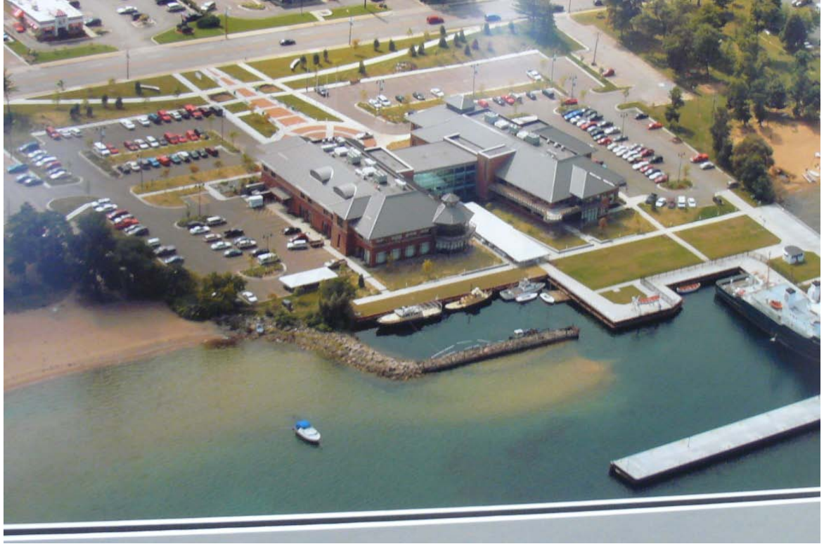
Figure 3. Aerial view of the NMC harbor illustrating the existing shoaling problem
