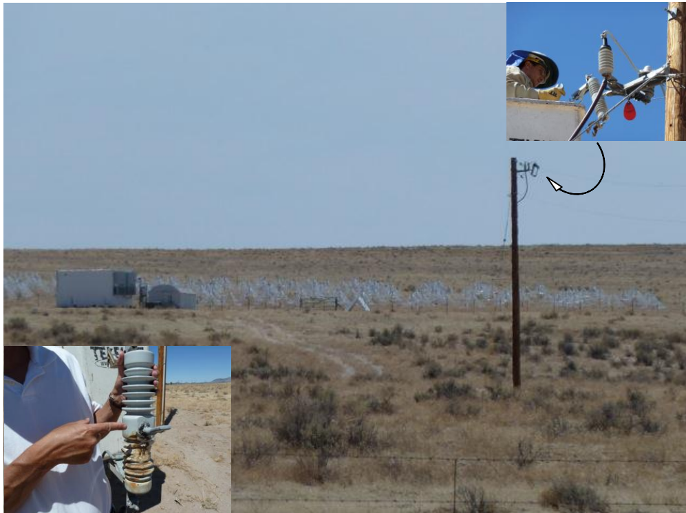
Figure 9: Identification of the source of the RFI in figure 8.
