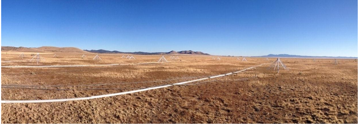
Figure 11: Antenna stands distributed over the outrigger site.
