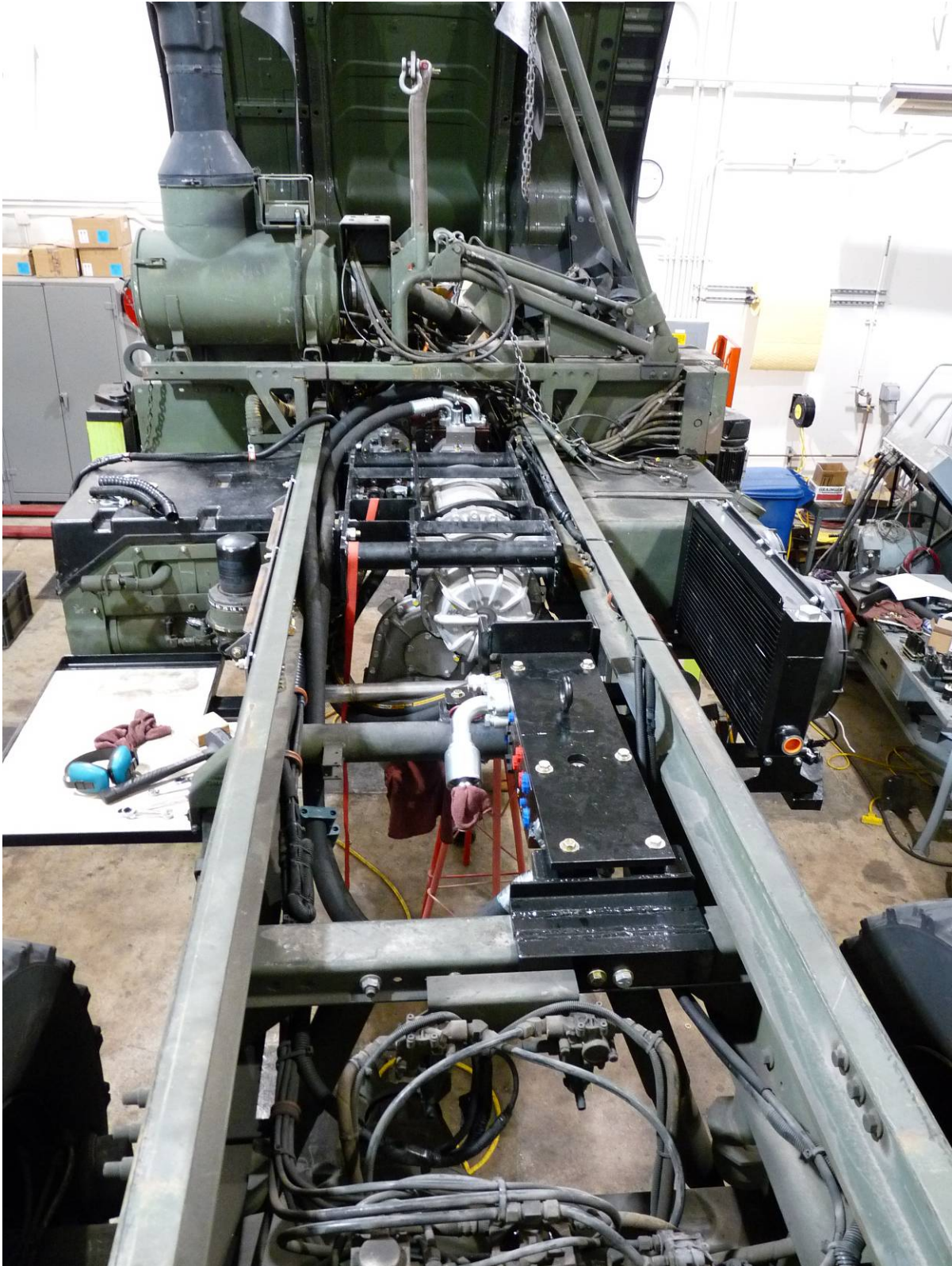
Figure 3.4.1-5. Installation of the Transmission and Drive Motor Assembly and the Megablock
