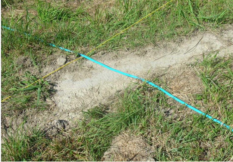
Figure 29 Copper Wire - 40 m Loops
