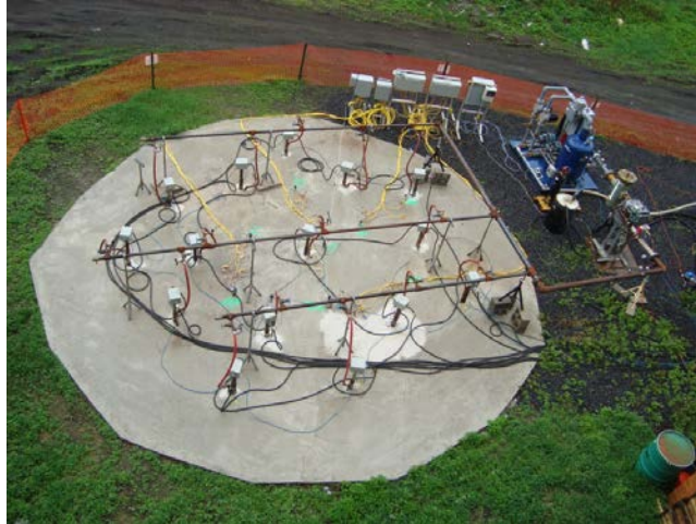
Figure 2-4 - Complete setup of the thermal conductive heating technology (TerraTherm, Inc.).
