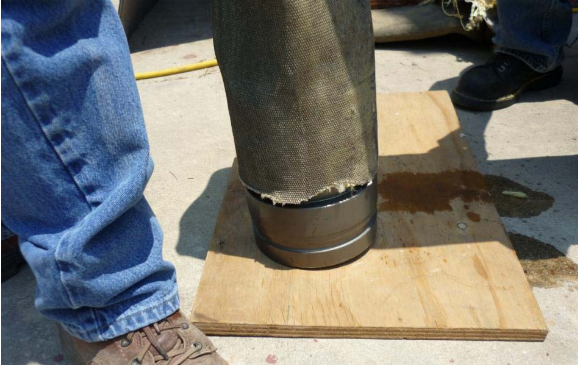
Figure 10. Inserting Shank into Conduit
