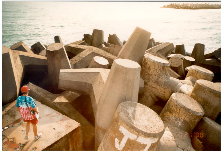
Figure 3. Head of Kahului west breakwater
