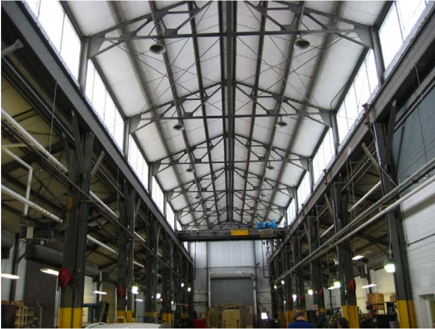
Figure 6. Mechanical Repair Shop.
