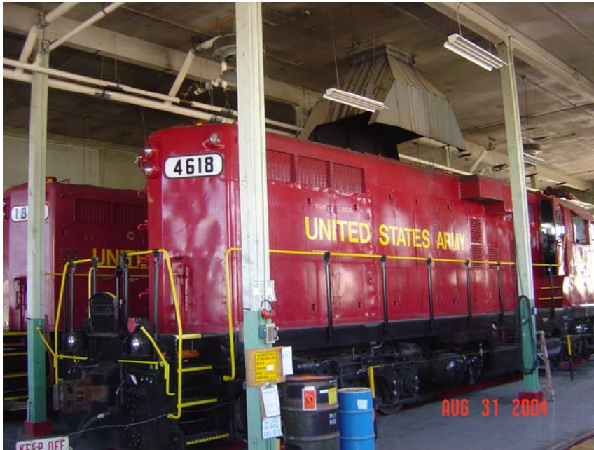
Figure 7. Locomotive Maintenance Facility.
