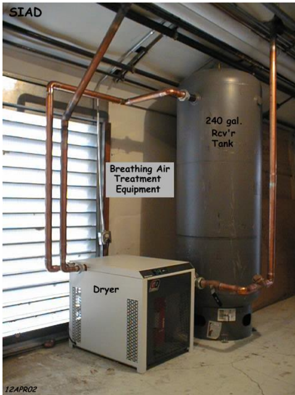
Figure 13. Oil-free compressor receiver and dryer.
