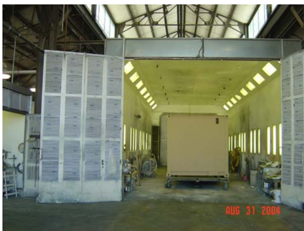
Figure 3. Drive-in spray booth in the Paint Shop.
