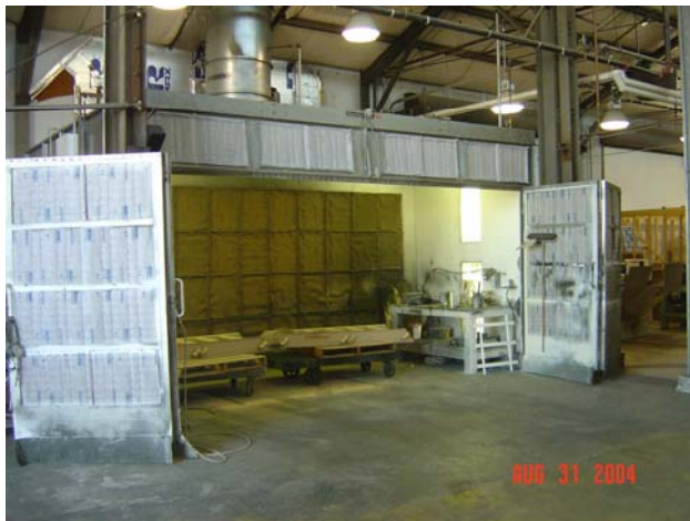
Figure 2. Spray booth in the Paint Shop.
