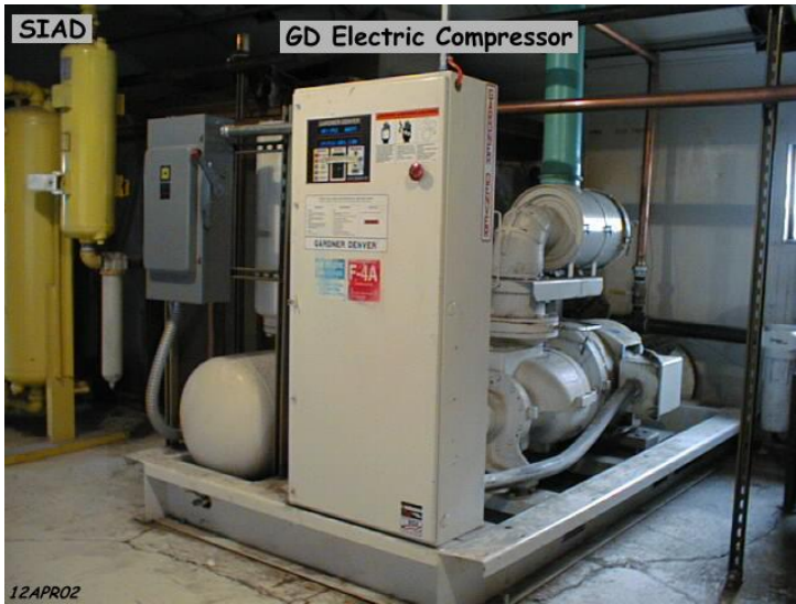
Figure 11. Backup Gardner Denver electric compressor.
