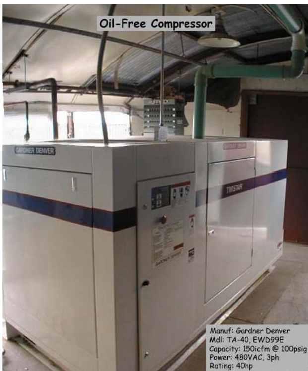
Figure 10. Gardner Denver TA-40 oil-free breathing air compressor.
