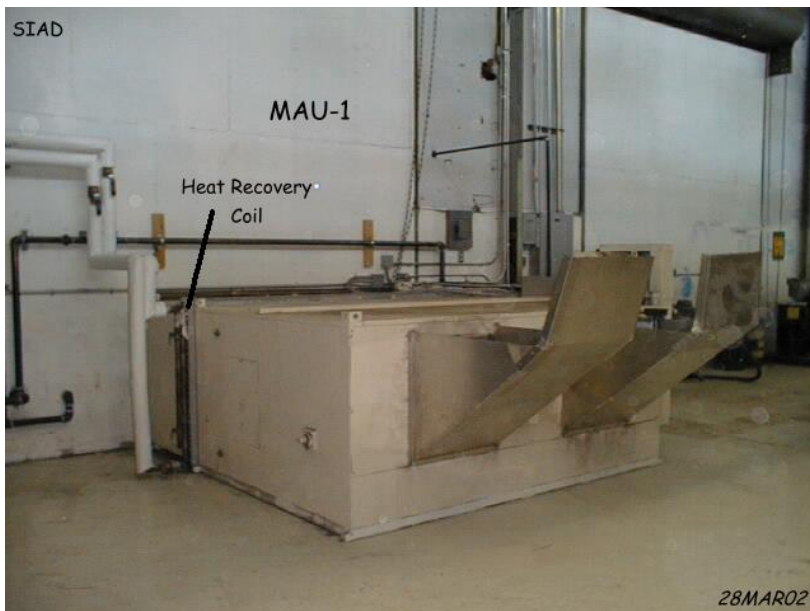
Figure 14. MAU-1 heat recovery coil.
