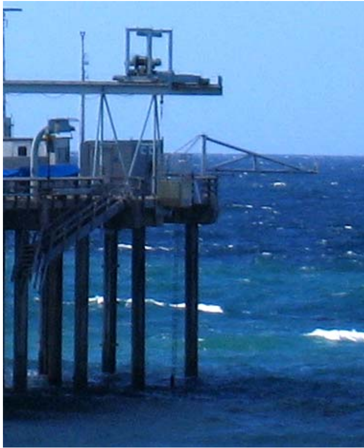
Figure 5: SIO pier showing the new boom off the NW corner.
