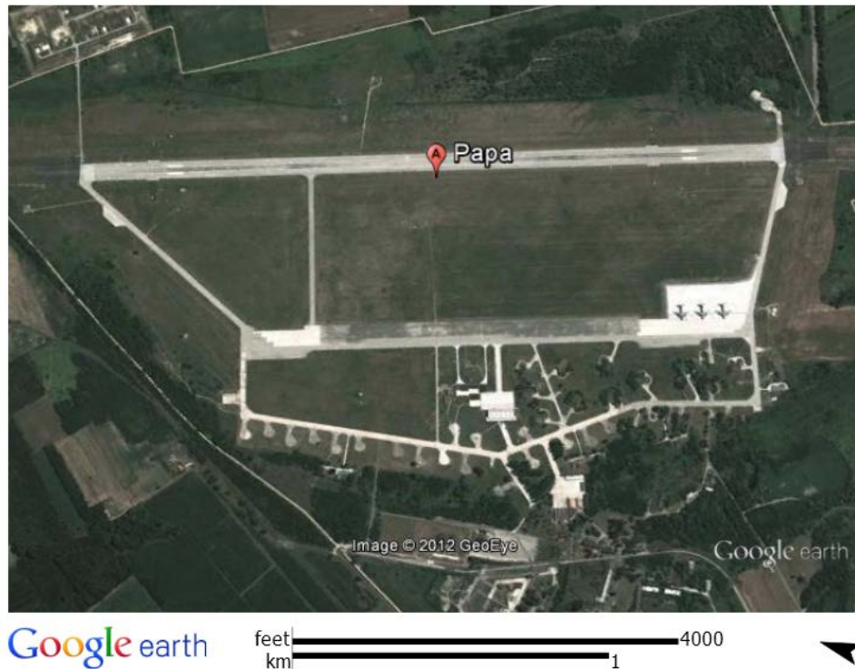
Figure 3. Aerial View of Pápa AB 69
