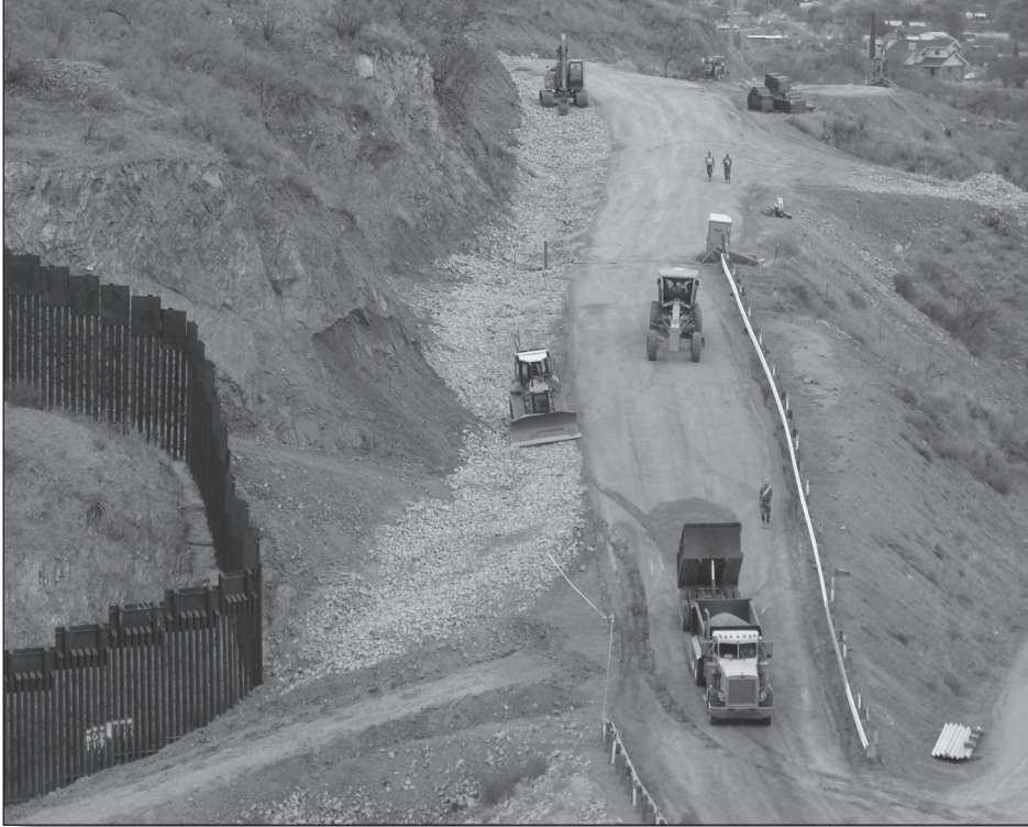
Navy Seabees construct an improved road east of Nogales, Arizona. To accomplish its engineer support missions along the Southwest border, JTF North employs engineers from all the military services.
