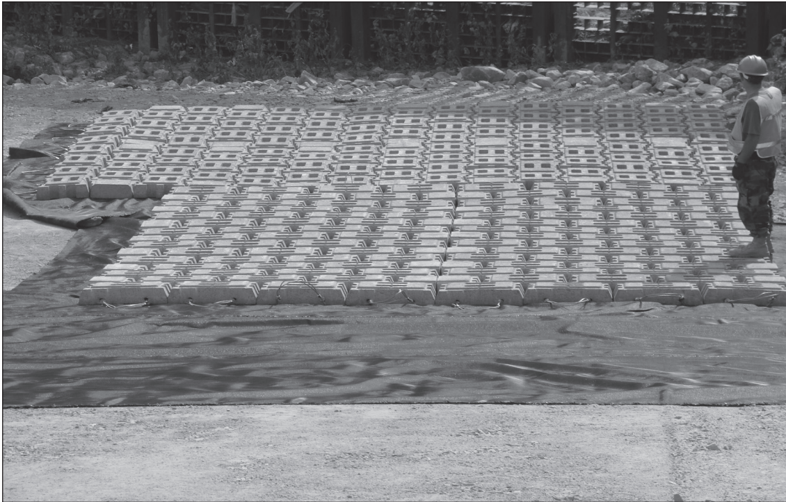
A Seabee observes the Armorflex installed for a low-water crossing along the United States–Mexico border. Reserve Component units use the JTF North engineer support missions to accomplish their annual two-week training requirement. Reserve Component units can rotate their personnel throughout the mission.
