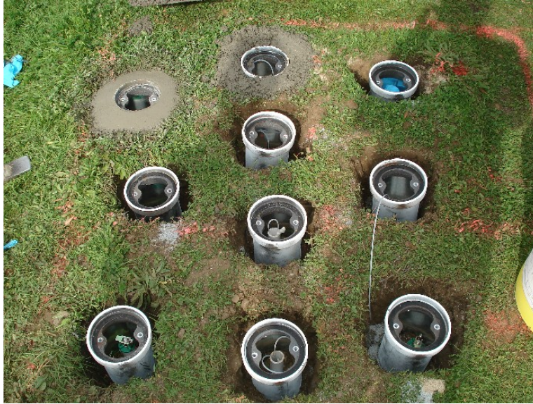
Photo 5.4.1: Example Soil Gas and Temporary Well Cluster (Travis AFB)
