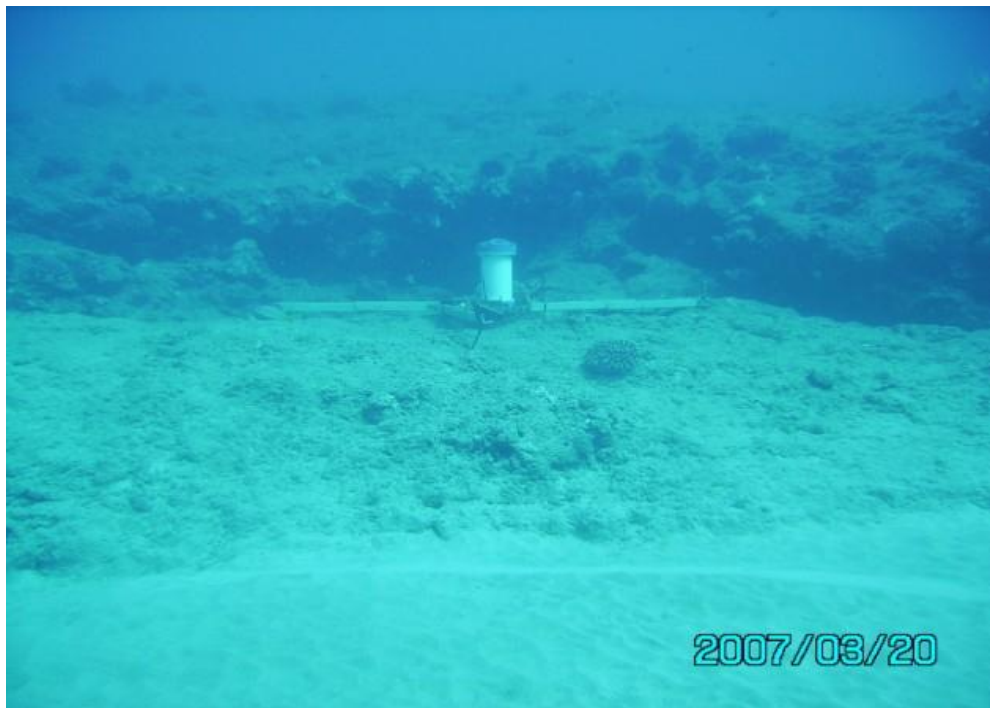
Figure 12. RD Instruments ADCP installed in the Offshore Field.
