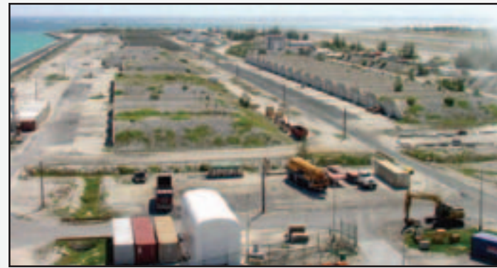
Chemical munitions were stored in bunkers in the Red Hat Area.
