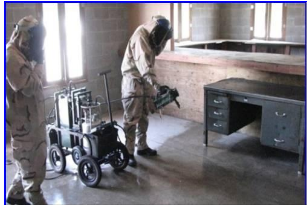
Figure 4-9. Indoor surface decontamination using the Peridox system.
