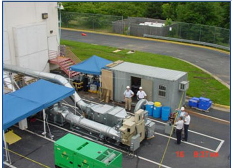
Figure 3-7. Decontamination activities at the Brentwood Postal Facility.
