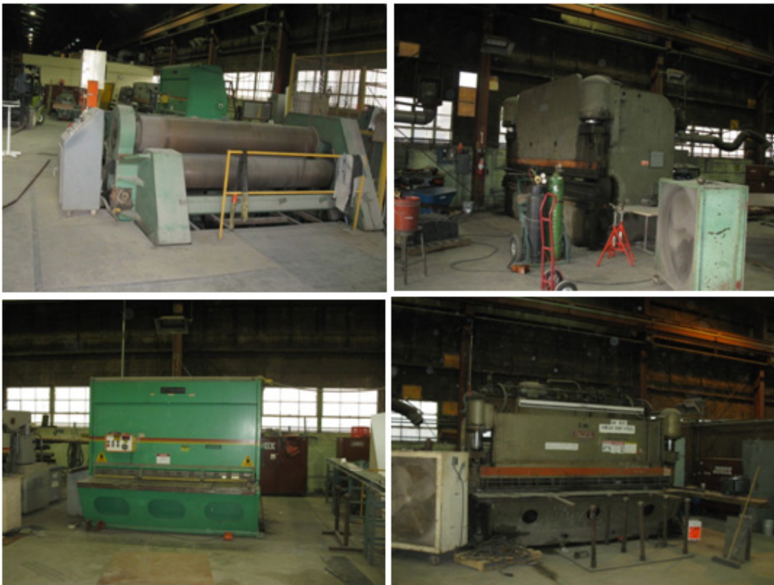
Figure 13. Various repair equipment at Ensley Engineer Yard.
