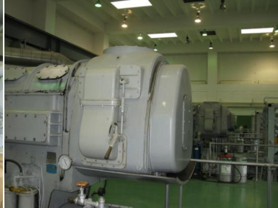
Figure 20. Diesel engine turbocharger.
