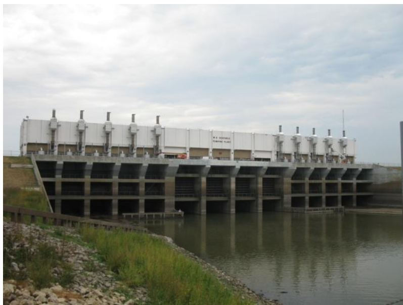
Figure 18. Huxtable Pumping Plant – downstream side.
