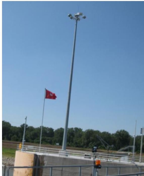
Figure 8. Mast lighting at Lock 27.
