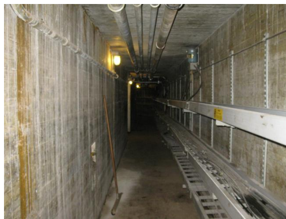
Figure 9. Lock 27 hallway lighting.
