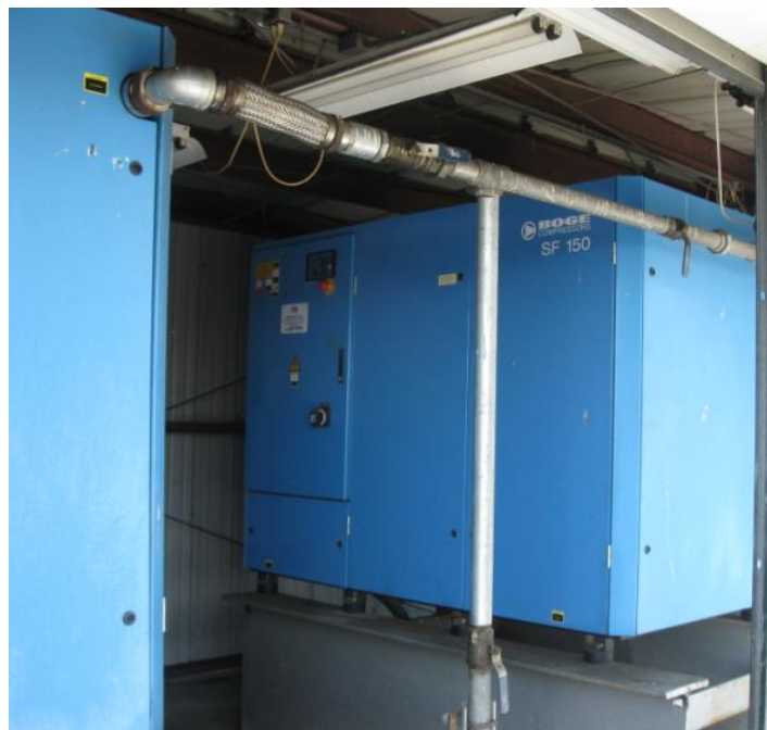
Figure 7. Lock 27 bubbler air compressor.
