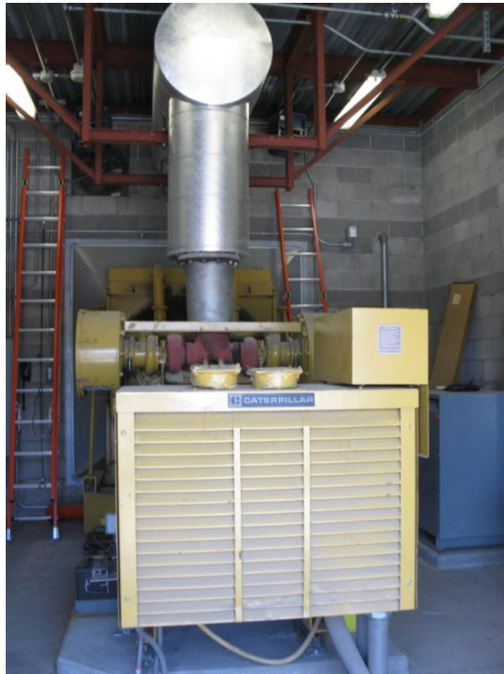
Figure 6. Lock 27 backup generator.
