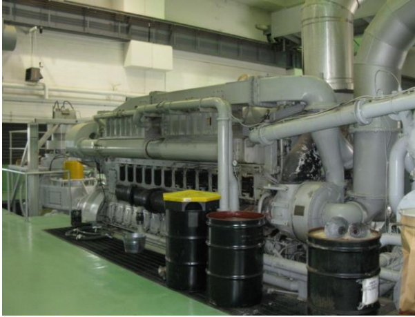
Figure 19. Fairbanks Morse 3600 hp diesel engine.
