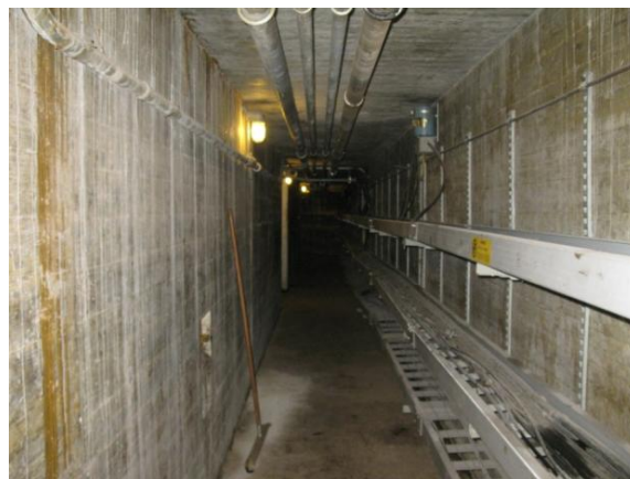
Figure 10. Lock 27 Lower hallway lighting.
