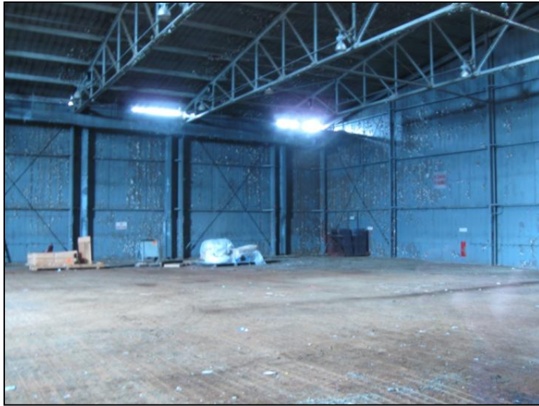
Figure 7. Interior view of the Air Force hangar.
