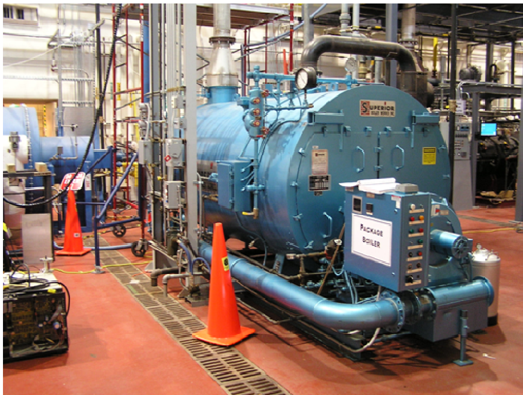
Figure 8-1. Marine package boiler at EPA facilities.
