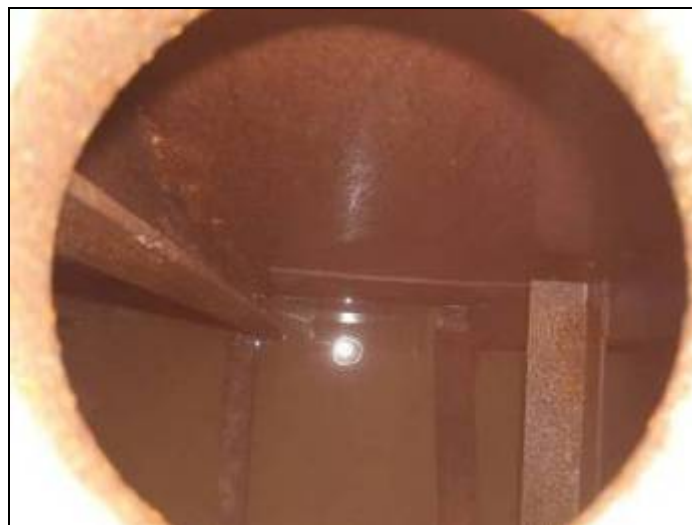
Figure 16. Typical tank inspection view.
