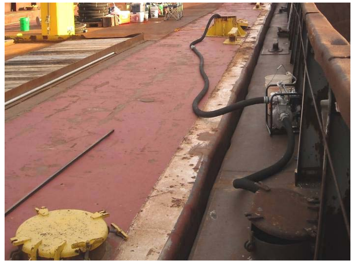
Pump and hose setup
