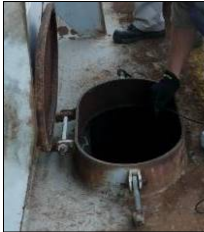
Figure 13. Ballast tank hinged manhole hatch.
