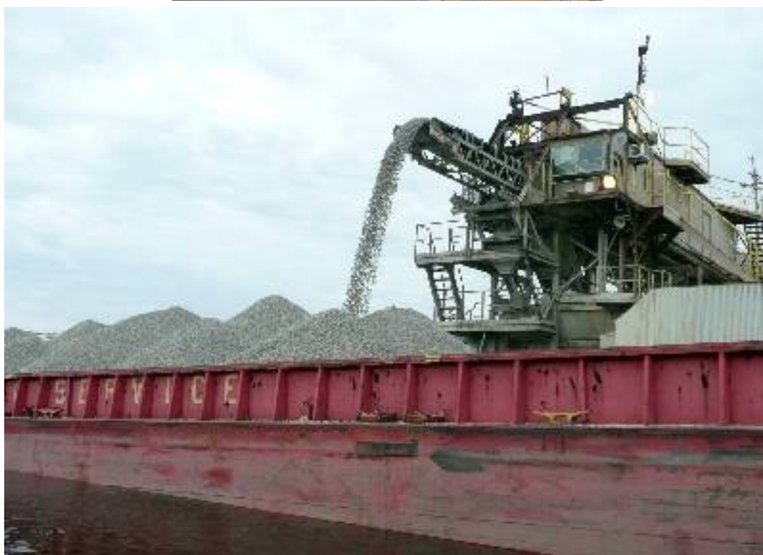
Figure C-2. Interior of empty hopper barge (upper). Loading hopper barge (lower).
