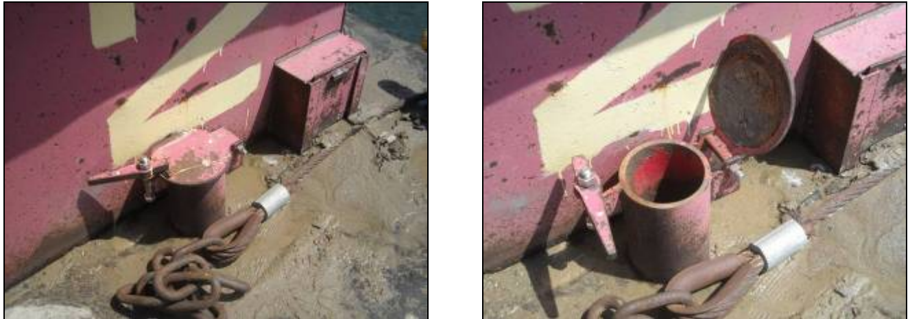
Figure 15. Ballast tank access tubes.
