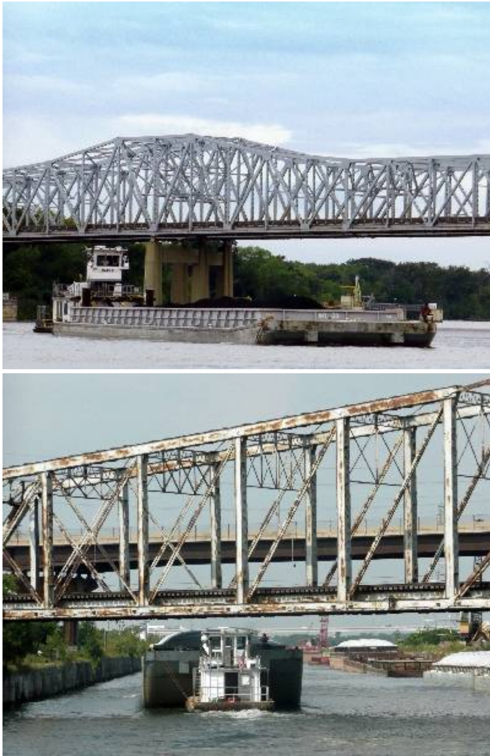
Figure C-1. Loaded (upper) and unloaded (lower) barges. Note minimal clearance under bridge.
