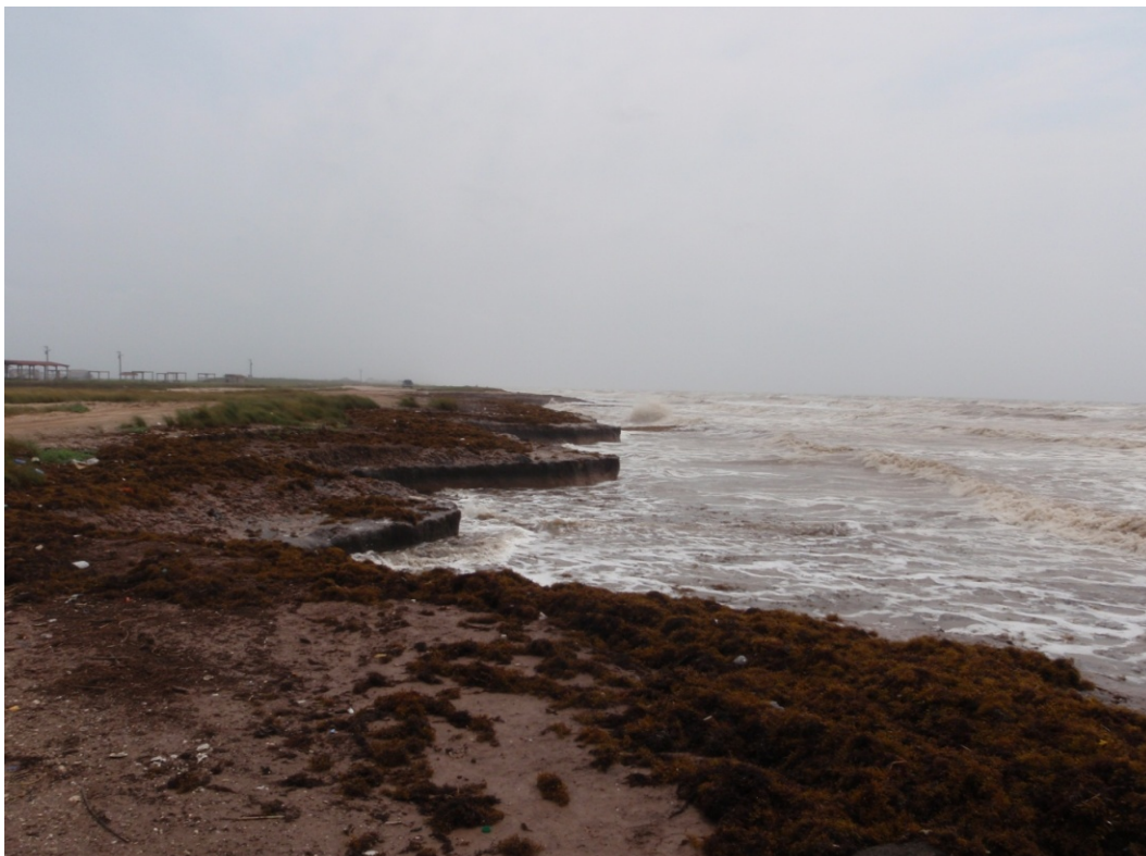
Figure 19. Sargent Beach near FM 457, facing northeast (May 2011).
