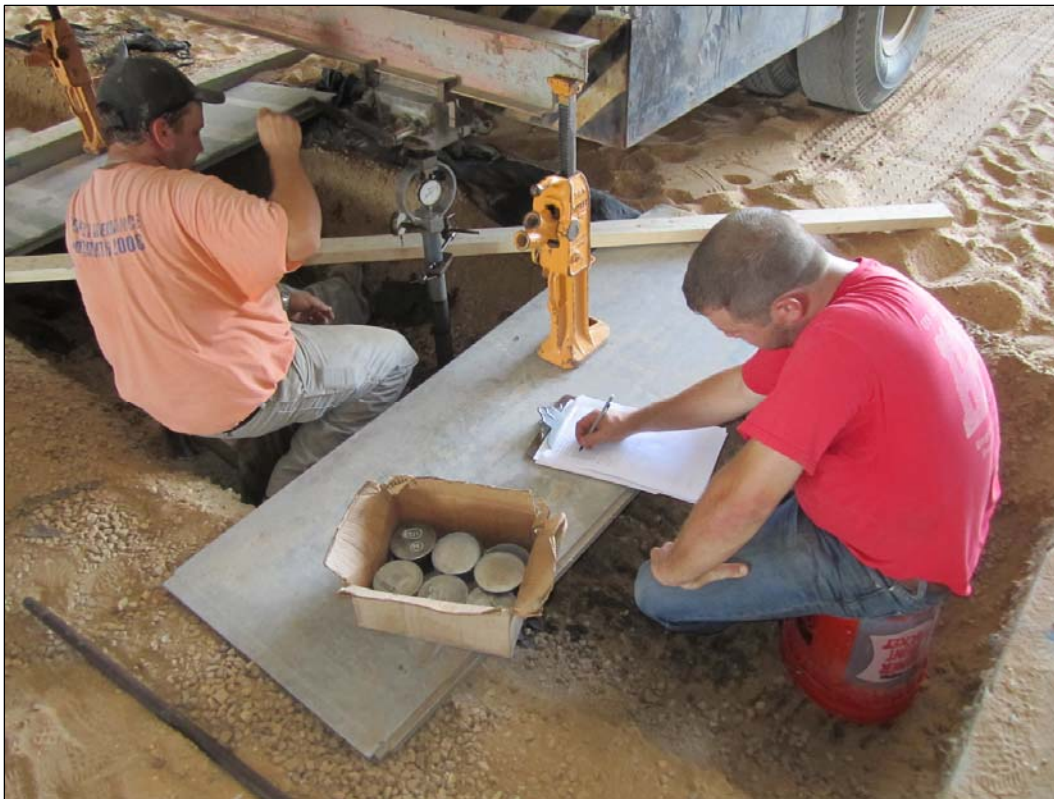
Figure 34. Subgrade CBR testing in trenched test item.
