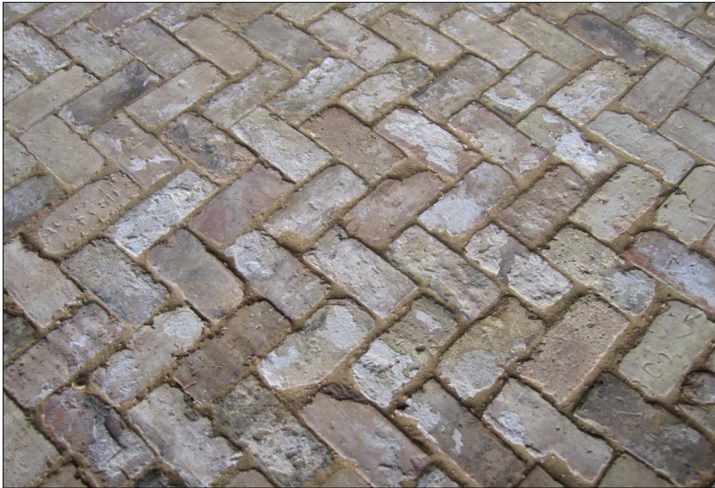
Figure 41. Reclaimed bricks before truck traffic.
