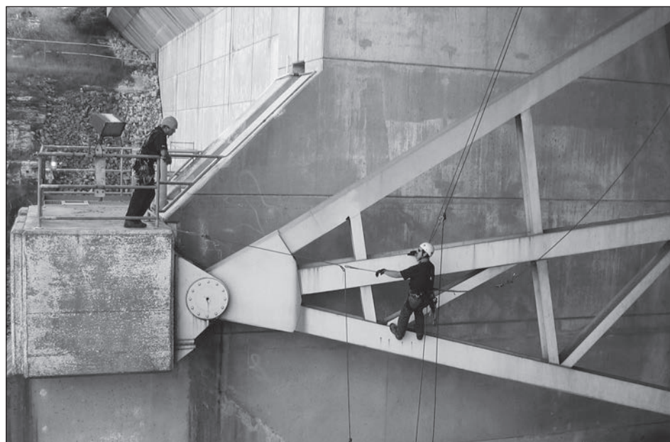
Technicians inspect one of four tainter gates on the Clarence Cannon Dam at Mark Twain Lake in Missouri.
