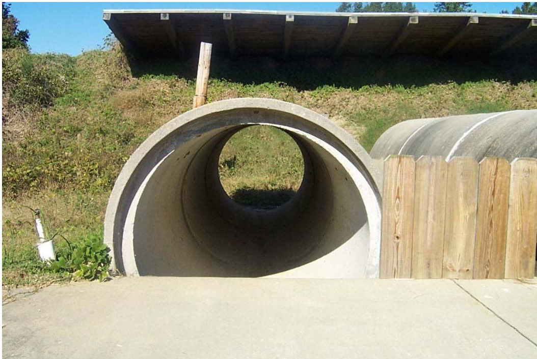
Figure 5. Pre-construction close up view through the pipe that forms the firing line and looking towards the berm.
