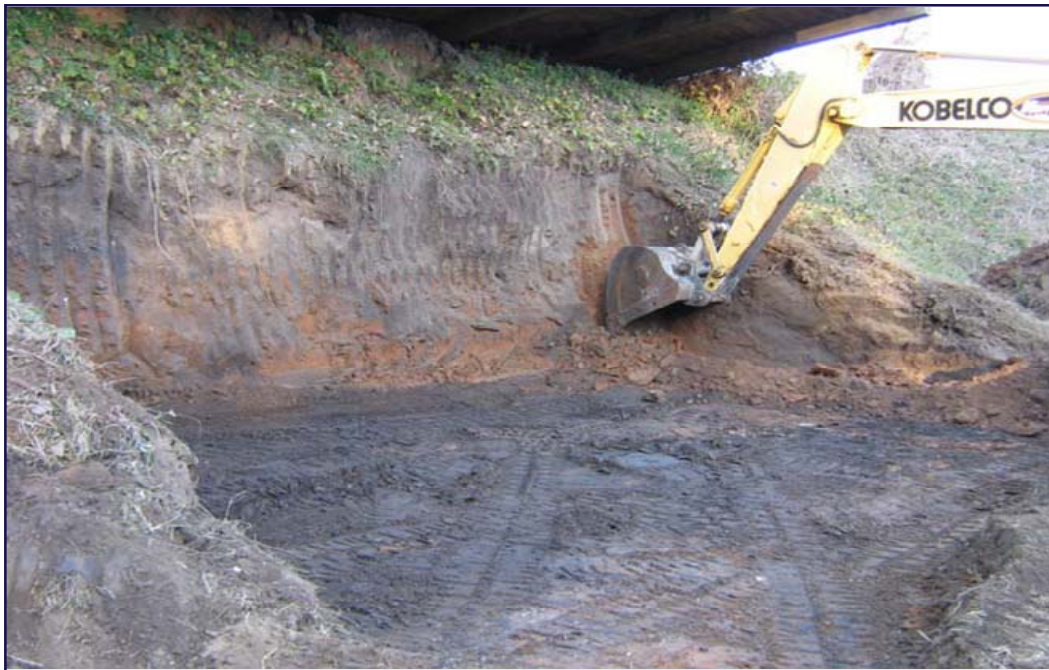
Figure 16. Removal of the old impact berm composed of local soil from under the newly constructed protective eyebrow.
