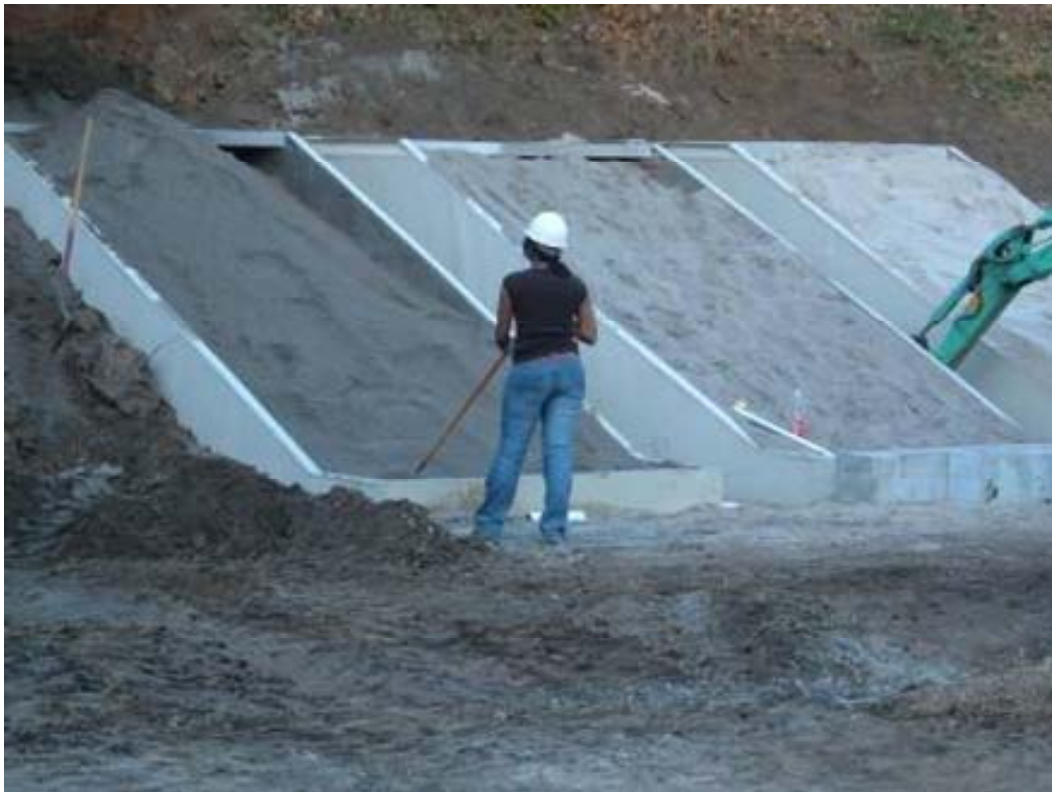
Figure 18. Placement of the amended ballistic sand in the lysimeters.
