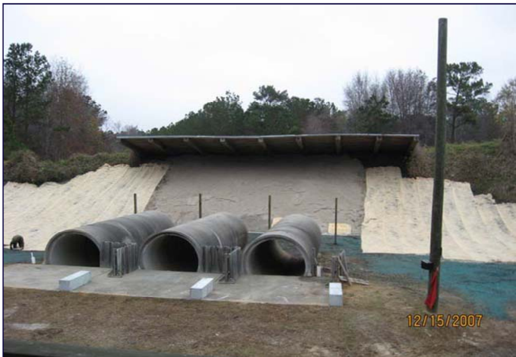
Figure 19. The completed impact berm enclosing the three experimental treatment lysimeters on the range, CAFB.
