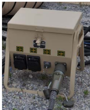
Figure 15. Power Distribution Panel (PDP)
