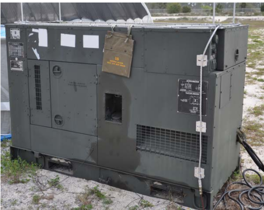
Figure 13. MEP-805A 30 kW Generator Figure 14. Secondary Distribution Center (SDC)
