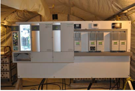
Figure 4. Component Panel Board (Front)
