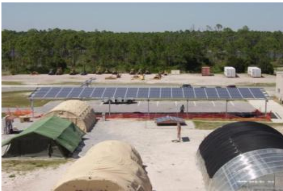
Figure 16. PV Array System Top
