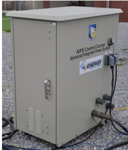
Figure 9. Data Acquisition Enclosure
