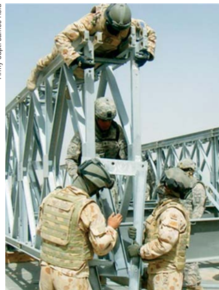
Australian and American combat engineers work to rebuild a bridge in Afghanistan.
