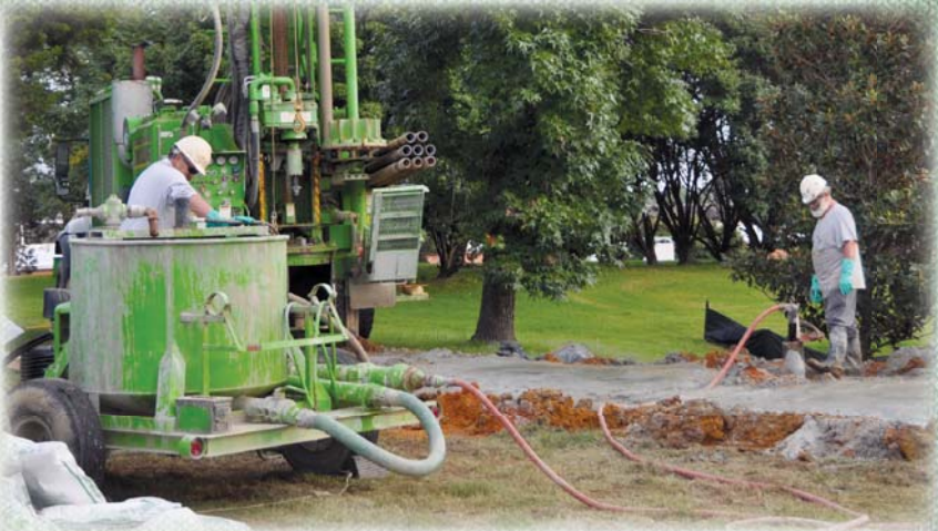
Contractors drill holes at Defense Supply Center Richmond, Va., for the installation of ground-source heat pumps. The new pumps are part of an energy-saving strategy to use about 50 percent less electricity than comparable air-source heat pumps.
