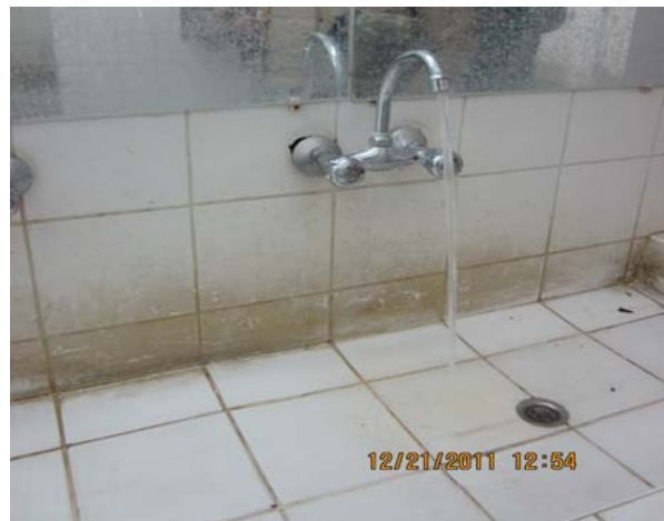
Figure 3 - Operational Sink in Latrine at Camp Hero, Kandahar
