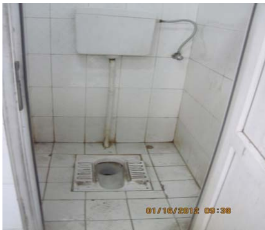
Figure 2 - Eastern Style Toilet in Good Repair in Latrine at Police District 3, Kabul
