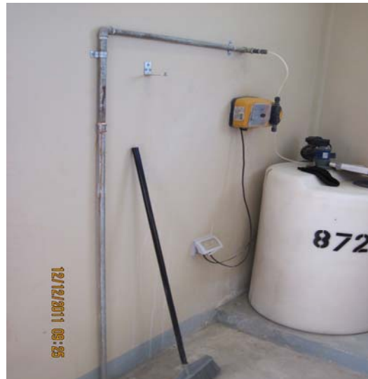
Figure 8 - Corroded Steel Pipe at the Joint Regional Afghanistan Security Forces Compound Water Treatment System
