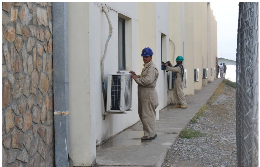
O&M trainees repairing heating and air conditioning units of barracks at the Kabul Military Training Center, SIGAR site inspection, October 2011.
