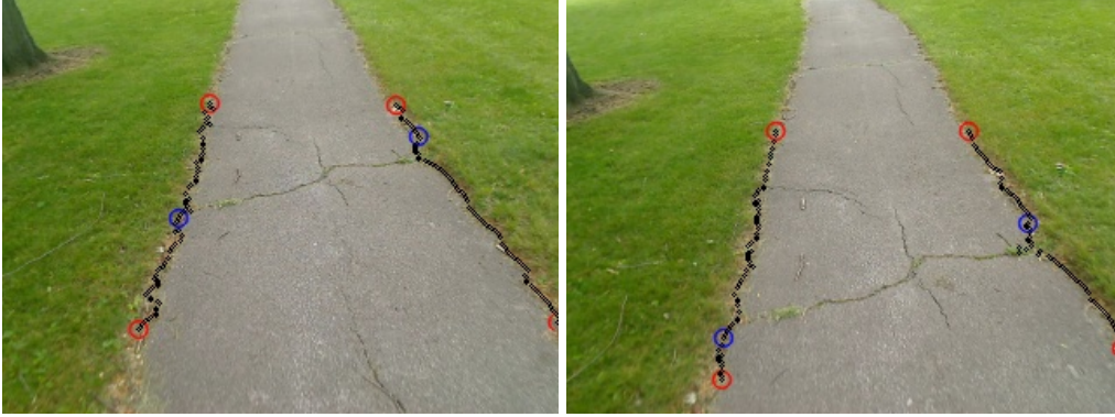
Figure 5.2: Early frame (left) and current frame (right), with measured curve endpoints for each frame in red and map curve endpoints in blue
