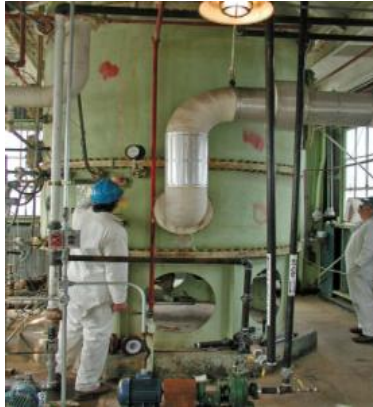
Construction of Solvent Recovery System underway
