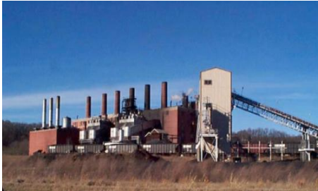
Current Holston AAP Coal Fired Steam Plant
