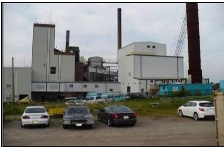
View of Iowa AAP's upgraded Coal Fired Steam Plant
