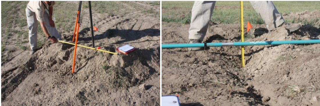
Figure 61. Surface Damage Failures, (left) Pile, (right) Hole
