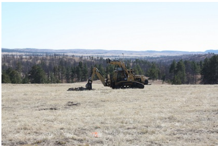
Figure 9. The ARTS on the Sub-Surface Range Digging for ISOs
