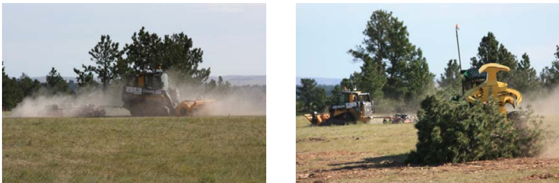
Figure 28. Team UXOD Skid Steer Mowing Task Operation
