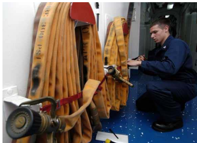
Figure 34. Firefighting Equipment Checks From [89]
