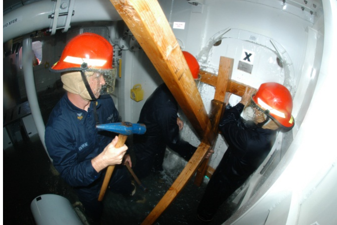
Figure 35. Damage Control Team Practicing K-type Shoring From [91]
