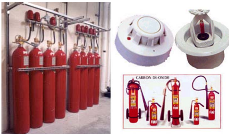
Figure 32. Wet and Dry Fire Suppression Systems From [88 (left), 89 (right)]
