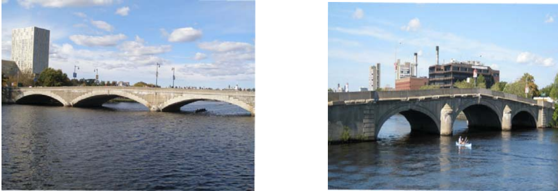
Figure 4: Western Avenue Bridge (left) and River Street Bridge (right)
