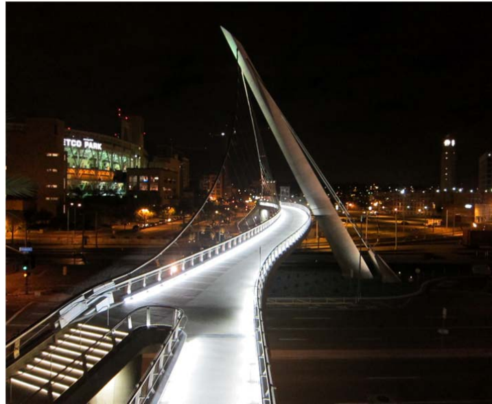
Figure 3: Harbor Drive Pedestrian Bridge
