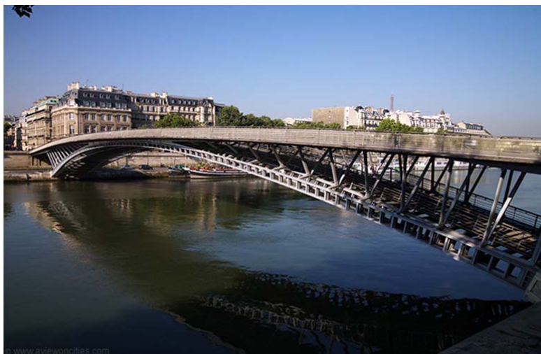
Figure 2: Leopold Sedar Senghor Bridge
