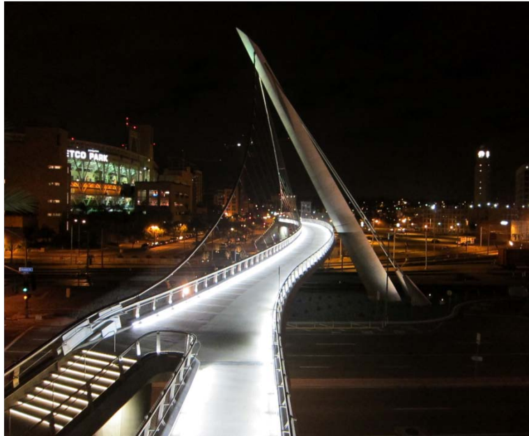
Figure 3: Harbor Drive Pedestrian Bridge
