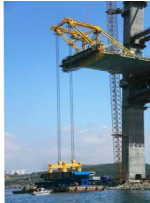
Figure 18: Deck installed by crane
