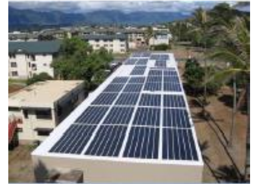
Rooftop PV K-Bay
