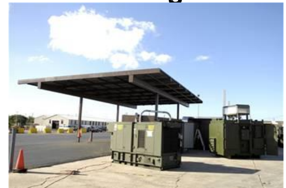
Hydrogen fuel station - Hickam
