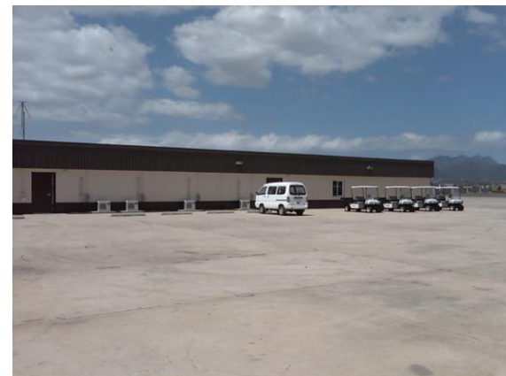
Guard bldg on Hickam with spray foam insulation on roof
