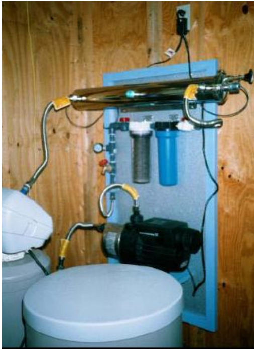
Disinfection array with pump, filters and UV lamp
