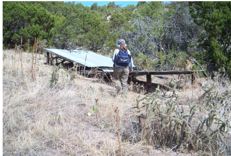
Figure 2. This rainwater harvesting system uses a prepared surface of concrete, rock or a sealing material to shed the rainfall. The rainwater is then diverted into the top of the collection tank
