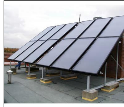
Flat plate solar collectors
