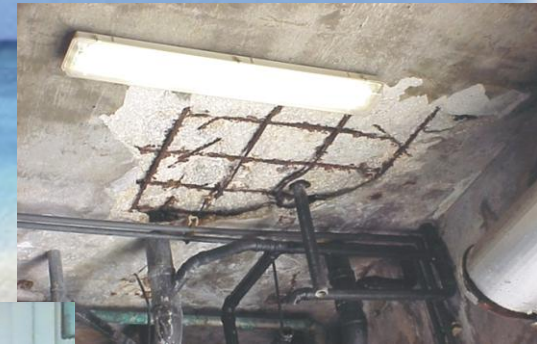
Spalling Concrete hazards
