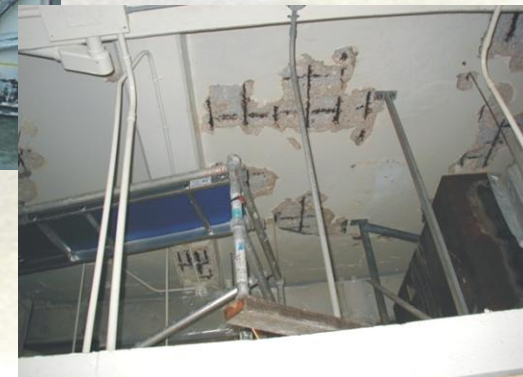
Spalling Concrete hazards
