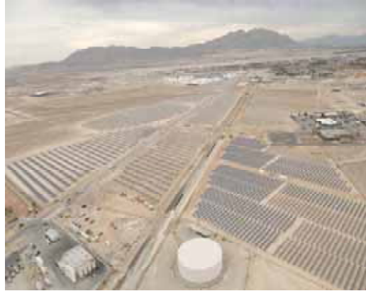
Photograph 1-1. SPVS at Area III on Nellis AFB constructed in 2007.
