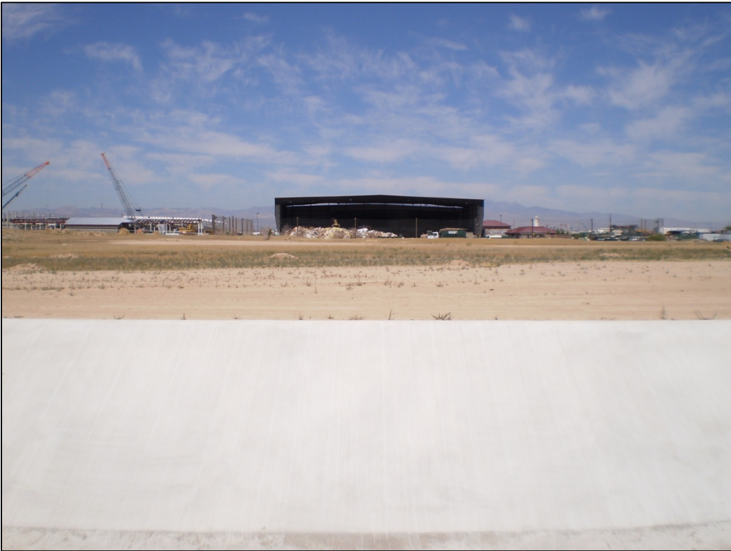
Photograph 1. West view from Sloan Channel
