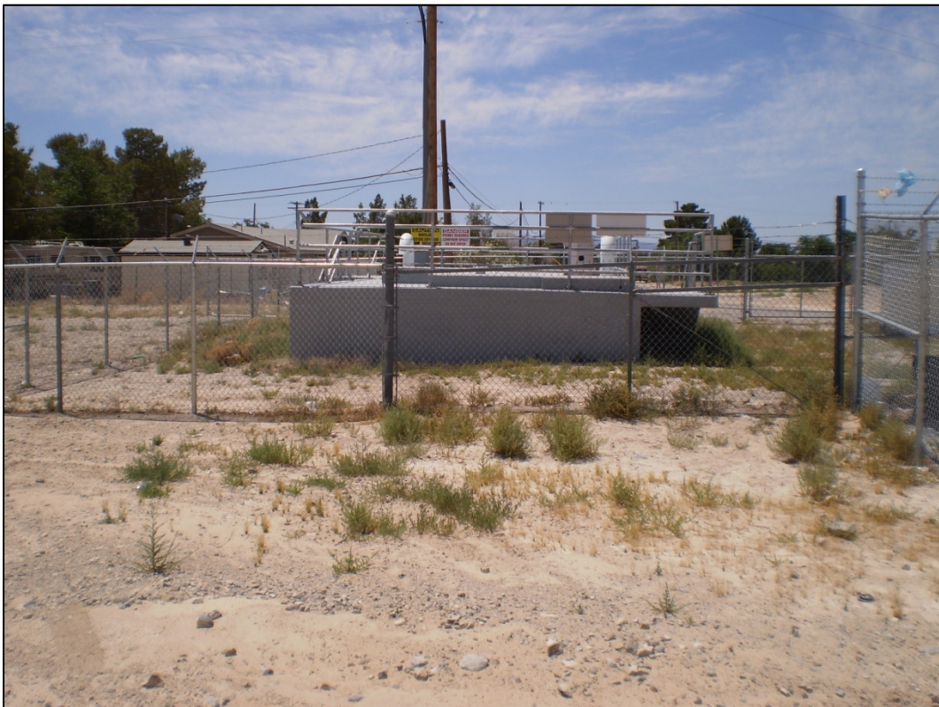
Photograph 14. Sewer pump station adjacent to the south property boundary
