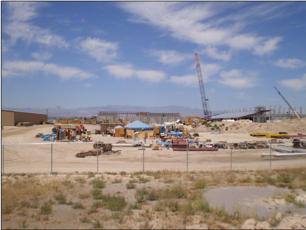
Photograph 17. Adjacent property to the west
