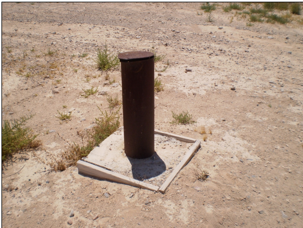
Photograph 12. Monitoring well at the southwest corner of the subject property
