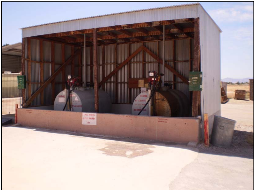
Photograph 18. ASTs in the golf course maintenance compound
