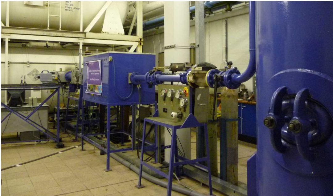
Fig. 5b HSST facility
