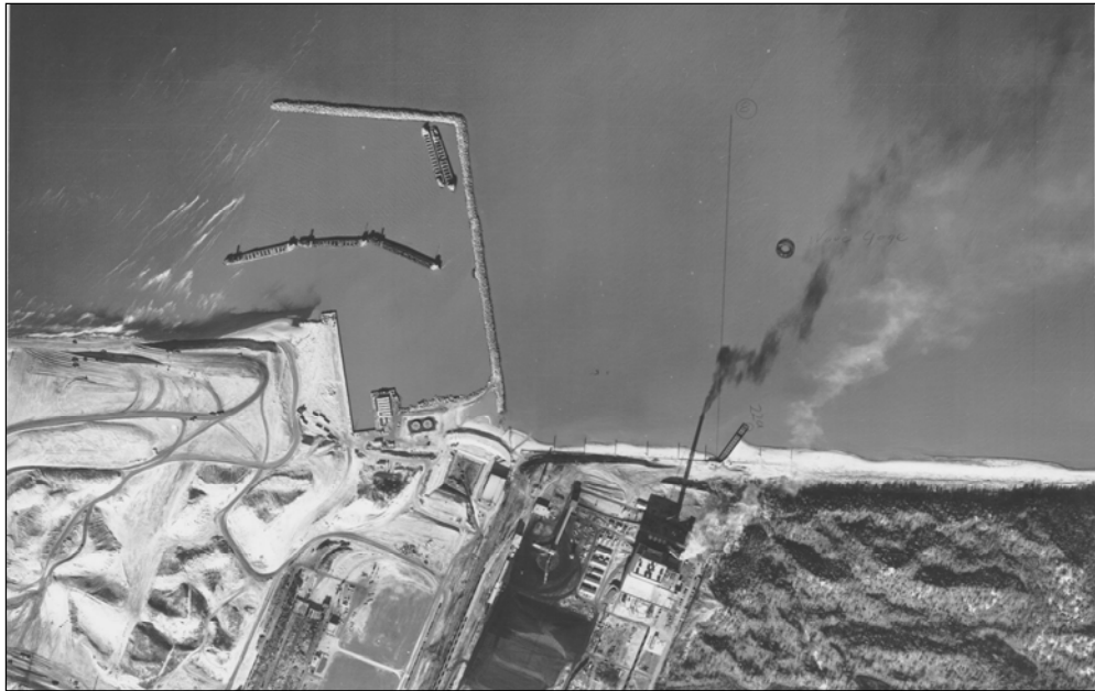
Figure 18. December 4, 1967. Bethlehem Steel (now Arcelor-Mittal) bulkhead construction is well along and the former dunes in the construction area have been mostly flattened. Shoreline configuration east of the bulkhead shows minimal change.
