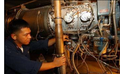
Allison 501k G/T Generator January 2011
