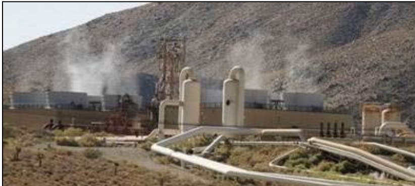
China Lake Geothermal Power Plant, 270 MW
