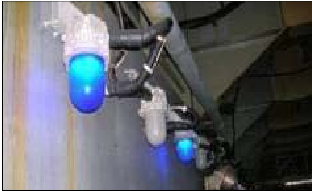
Efficient Ship Systems Example: Solid State Lighting
