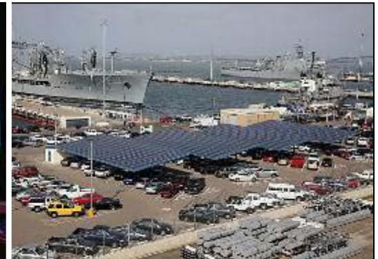
San Diego Solar PV
