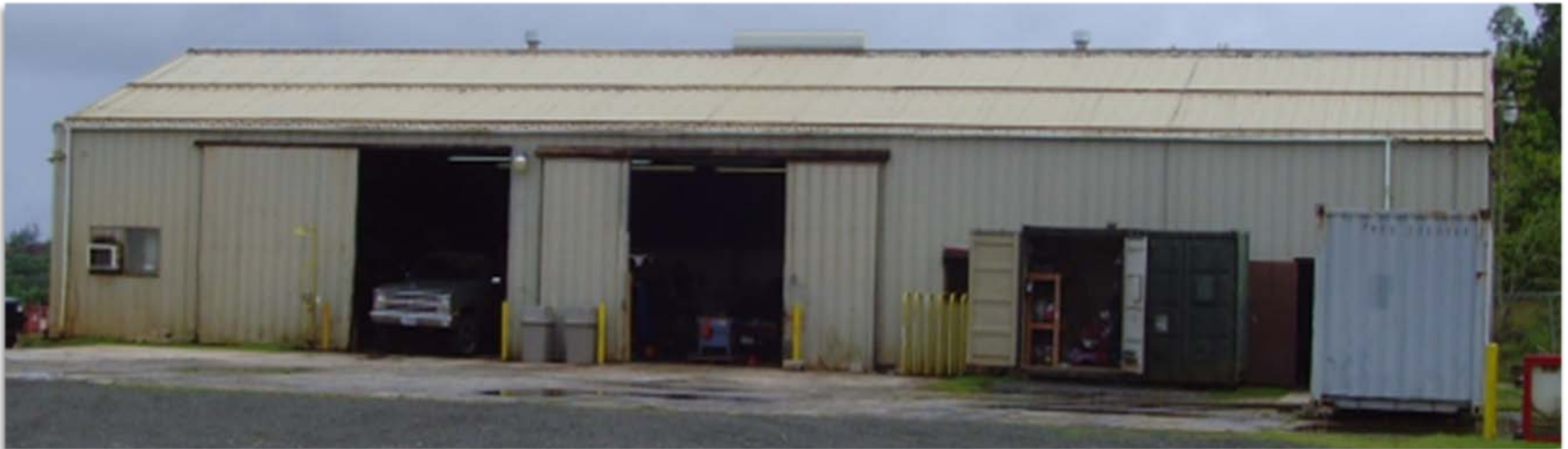
Camp Katuu Builder's Shop – PV Array Installation Location
