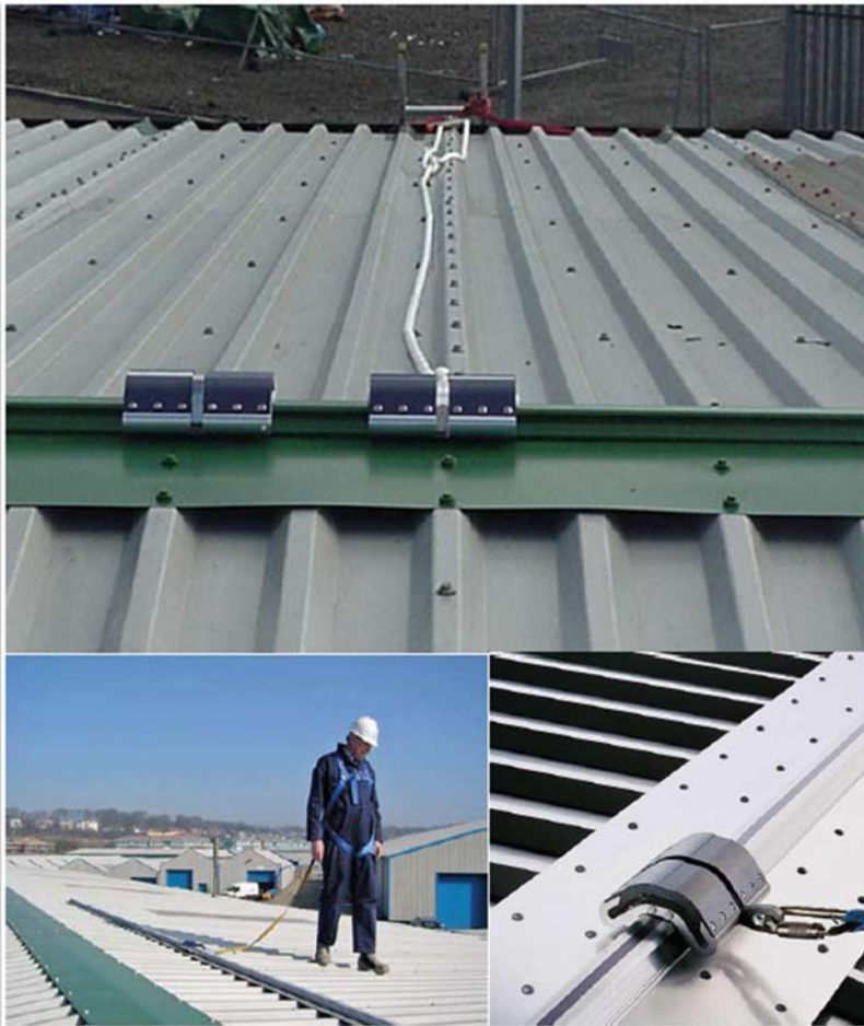
Figure 7: Rail Type Fall Protection System
