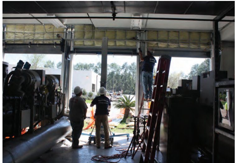
Installation of a pair of cost-saving, high-efficiency 700-ton magnetic chillers begins
