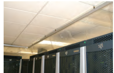
Containment enclosure installed to block airflow over tops of system cabinets
