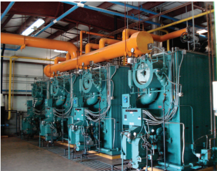
Figure 3.6 Fort Knox Hospital Boilers
