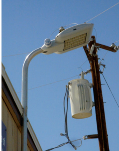
Figure 3.2 Fort Irwin Experimental LED Street Light
