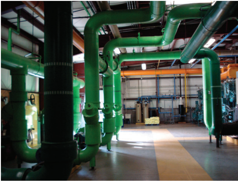
Figure C.7 Fort Knox's Hospital Chilled Water System
