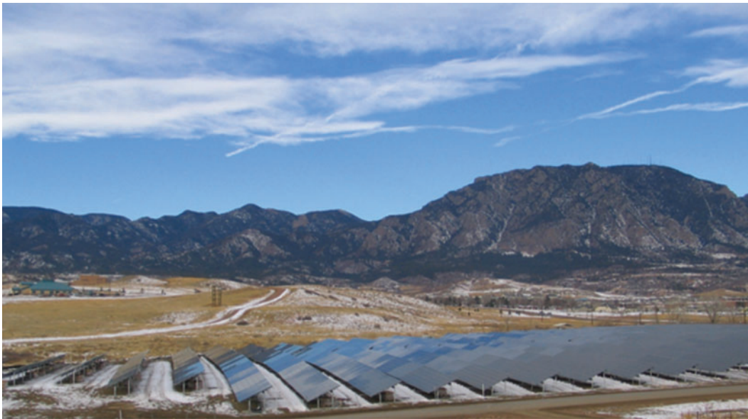
Figure 2.2 Fort Carson Two-MW Solar Array
