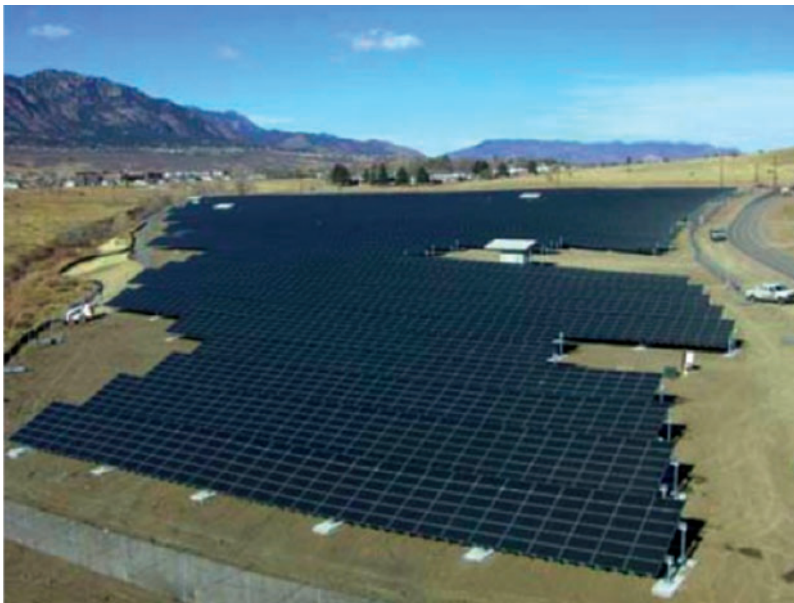
Figure B.5 Fort Carson Two-MW Solar Array
