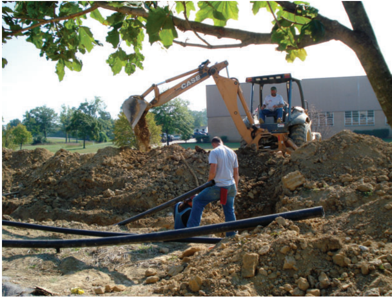
Figure C.5 GSHP System Being Installed at Fort Knox
