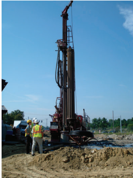
Figure C.4 Drill Rig Being Used to Dig GSHP Wells at Fort Knox
