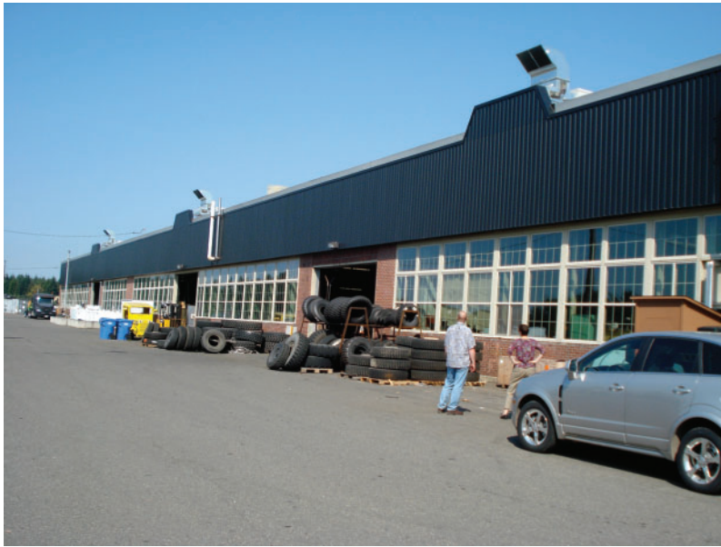
Figure D.1 Fort Lewis SolarWall on a Logistics Warehouse
