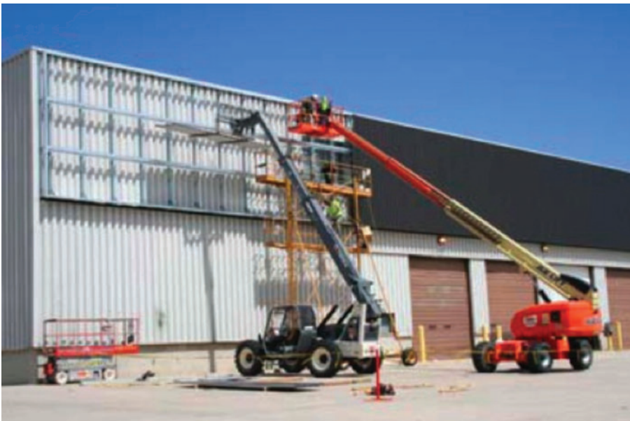
Figure B.6 Installation of Fort Carson Solar Wall
