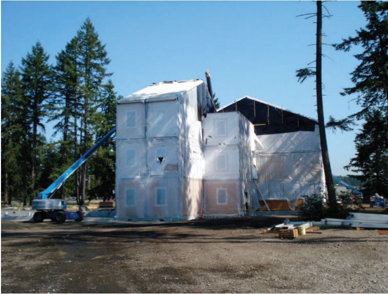
Figure D.2 Modular Building Construction at Fort Lewis
