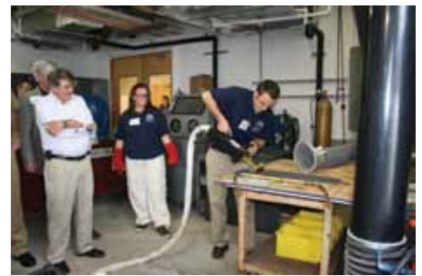
Demonstration of the removal of non-skid coating by heat induction at NRL Key West.
