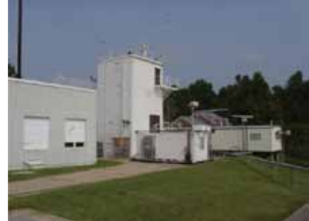
The Chesapeake Bay Detachment Radar Range facility overlooks the shipping channels in the Chesapeake Bay, in conjunction with the extensive Marine Navigation Radar (MNR) Test Range on Tilghman Island.
