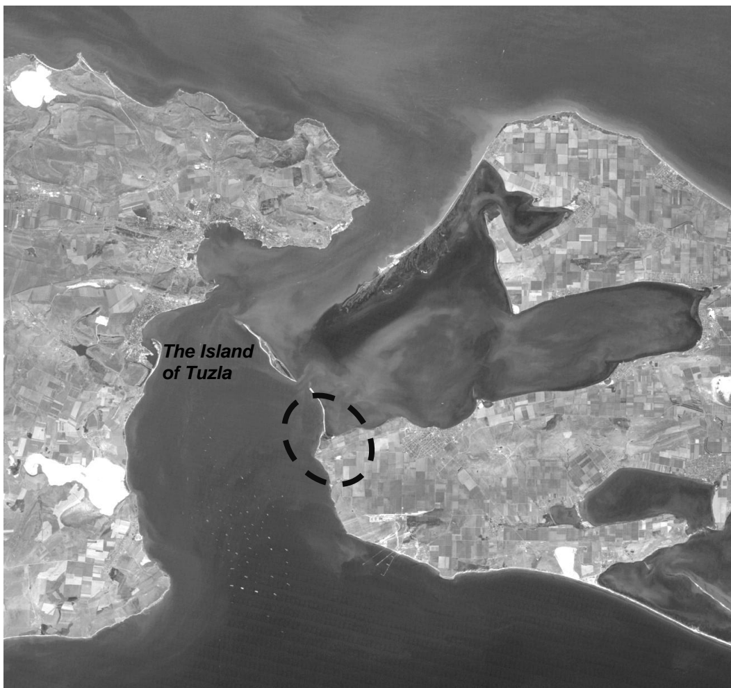
Figure 2. The dam constructed in the Kerch Strait.
