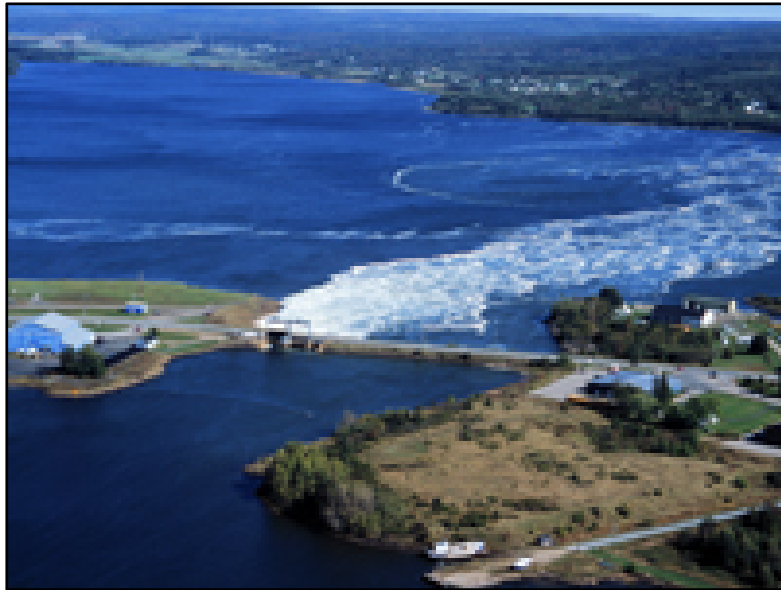
Figure 1 Annapolis Tidal Power Plant in Nova Scotia, Canada (From [4])
